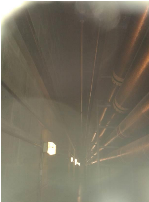
Level 1 service duct adjacent to former parcels office – looking north
