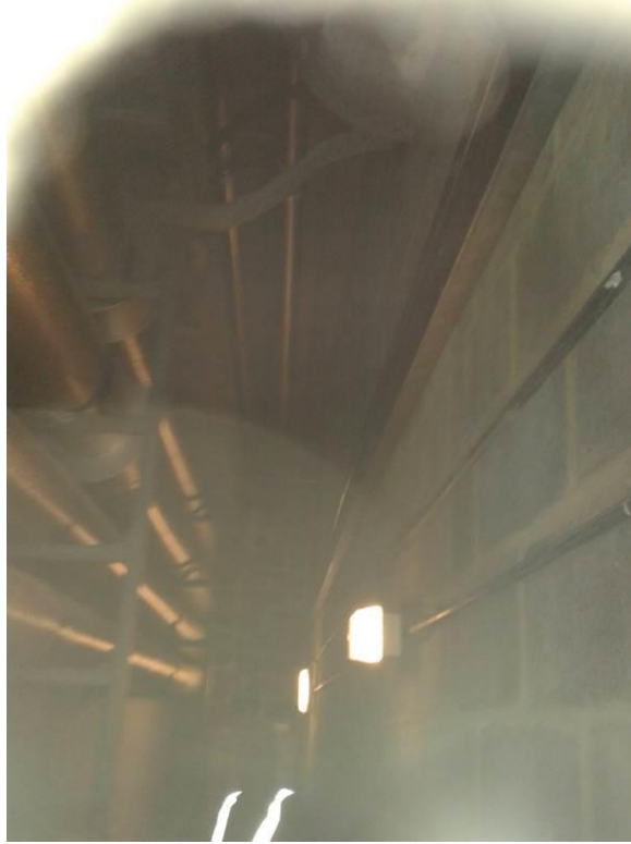
Level 1 service duct adjacent to former parcels office – looking south
